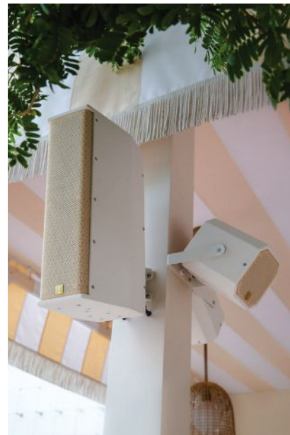
At left, Panorama MS34 loudspeakers deployed in mono+stereo mode deployed in one of the cabanas, while at right, a Tower LCC44 and Cannon C4 address specific coverage zones.
